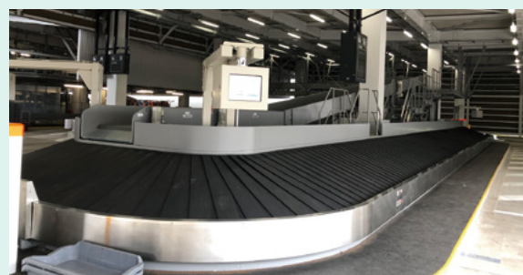
South Wing of Narita International Airport's Terminal 1
