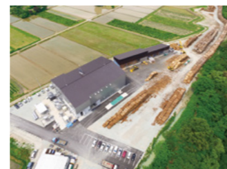
Woody biomass gasification plant
