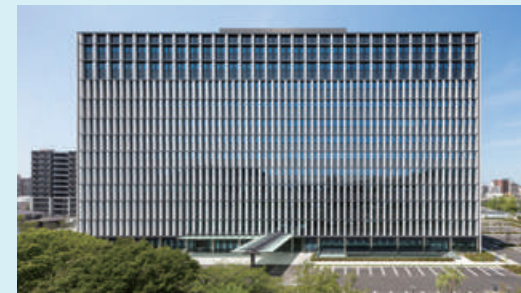
Fukuoka High Court, District Court, Family Court and Summary Court building
