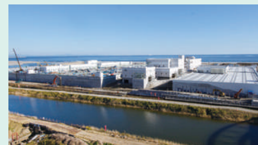
Minami-Gamo Purification Center
