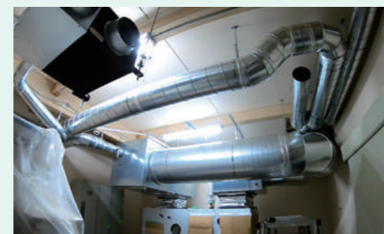
Construction work around the air conditioner in the machinery room of the Basic Observation Building
