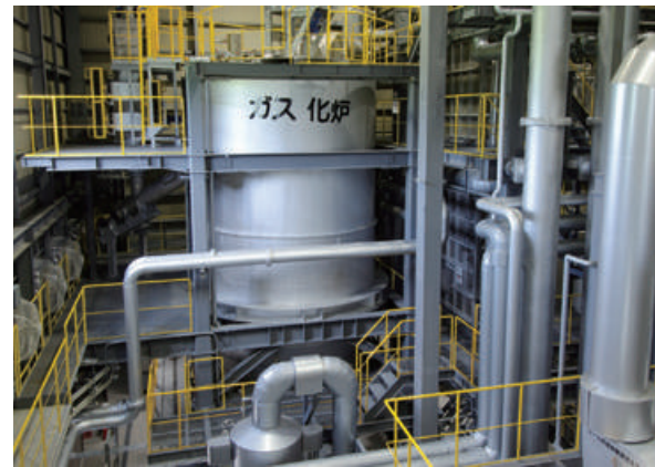
Woody biomass gasification power generation facility of NKC Nagai Green Power Co., Ltd.
