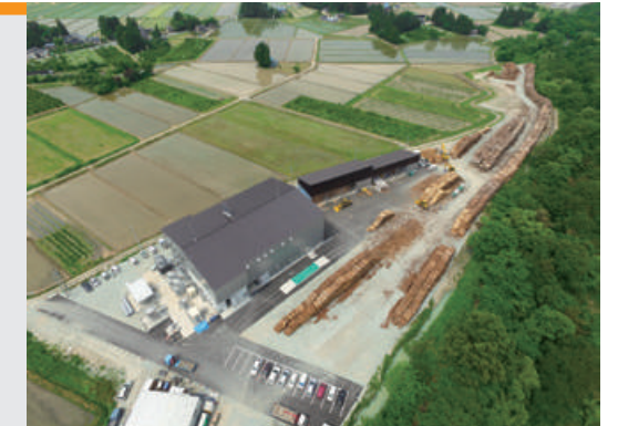
Woody biomass gasification power generation plant of NKC Nagai Green Power Co., Ltd.
