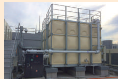
Elevated tank for recycled water
