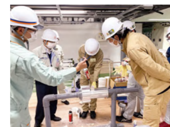
Technical skills training by a subcontractor
