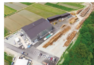
Woody biomass gasification plant
