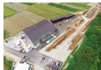
Woody biomass gasification plant
