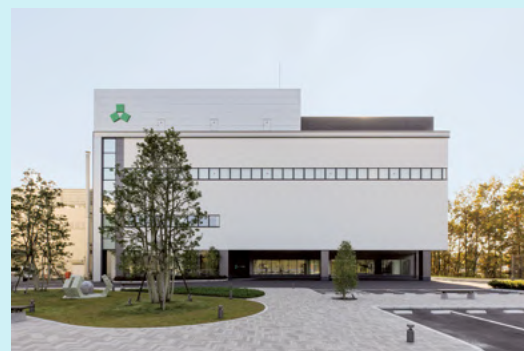
Kanae Tochigi Factory No. 3 Factory Building
