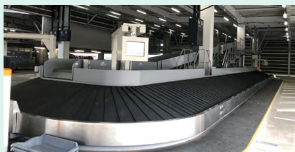
South Wing of Narita International Airport's Terminal 1
