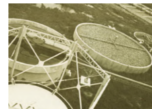
Night-soil treatment plant
