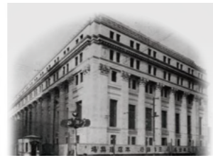
Mitsui main building
