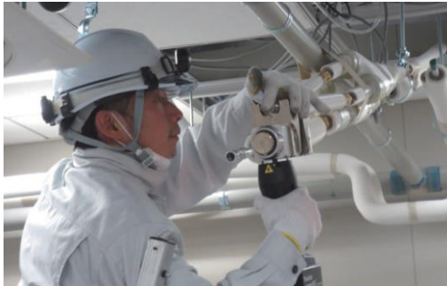
Market rollout of aluminum refrigerant piping method “Aluminger”
