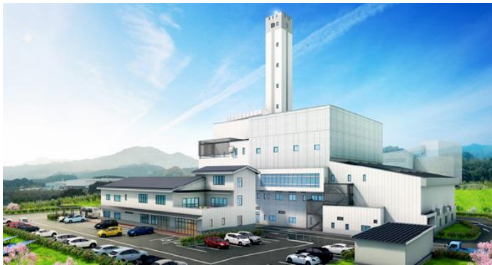
Received first order for DBO style of energy-recovery waste treatment facilities including new construction work(Saga Prefecture)
