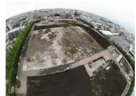
Scene of the demolition of the old Yamato Plant
