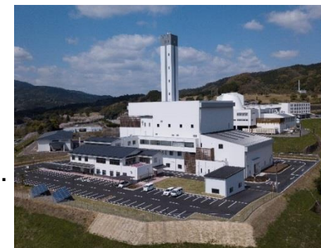
Exterior of Clean Hill Tenzan
