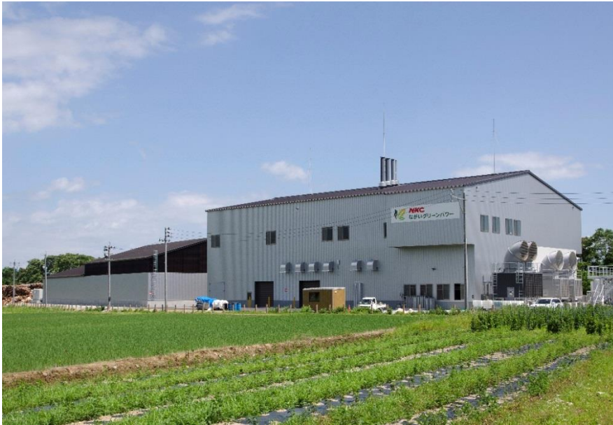
Exterior of plant building
