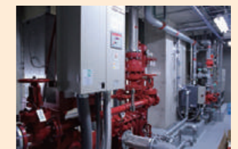
Sprinkler pumps installed on the second basement floor
