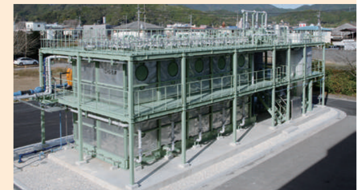
Demonstration facility at the wastewater treatment plant in Susaki City, Kochi Prefecture
