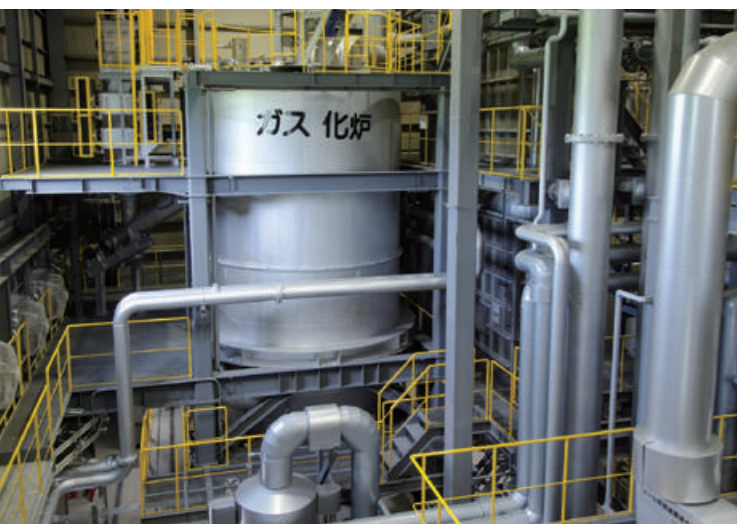
Woody biomass power generation plant of NKC Nagai Green Power
