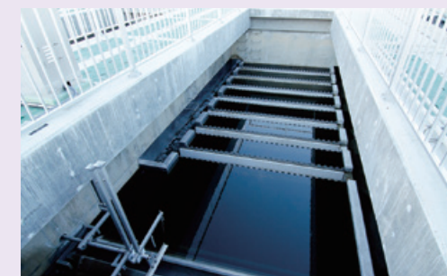
Final sedimentation tank
