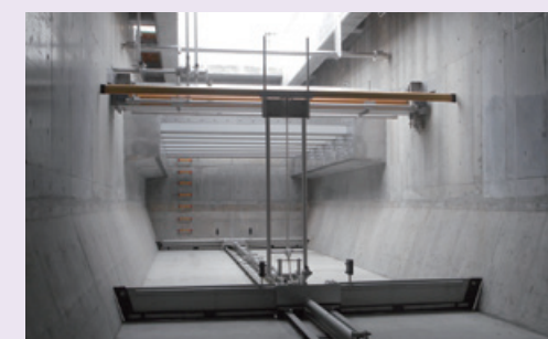
Monorail sludge collector
