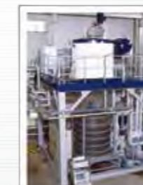
Ice thermal storage system
