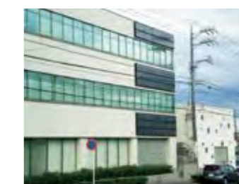
Solar generation at the Toyota branch facility
