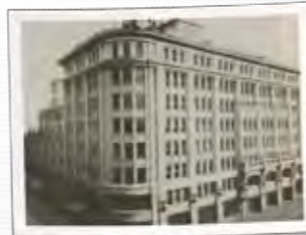
The Nihon Seimei Building, Tokyo
